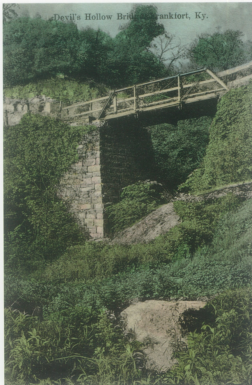
Fr 20 - Devil's Hollow Bridge, Frankfort, Ky.
